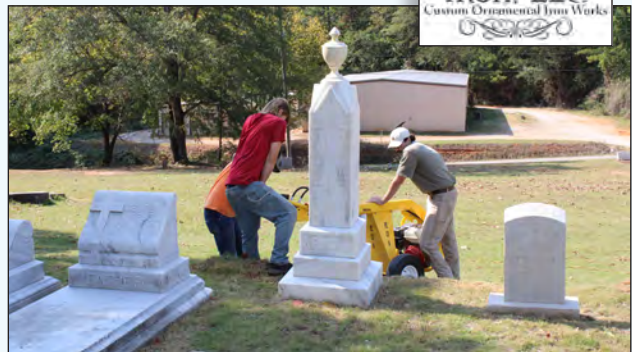
A compact motorized auger needed some pressure from the three man team but it did a fine job of "punching" holes for the fence posts in the rock-hard ground of Montevallo City Cemetery.
