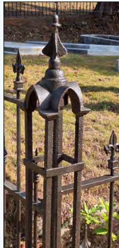
(Left) To the surprise of many, the sturdy original iron corner posts could be restored and re-used in the new configuration. (Right) A brass gate latch handle, with a patina of "verdigris" was resurrected by Ensley Iron and reused.
